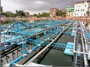
Floating Fountains Installation Service
